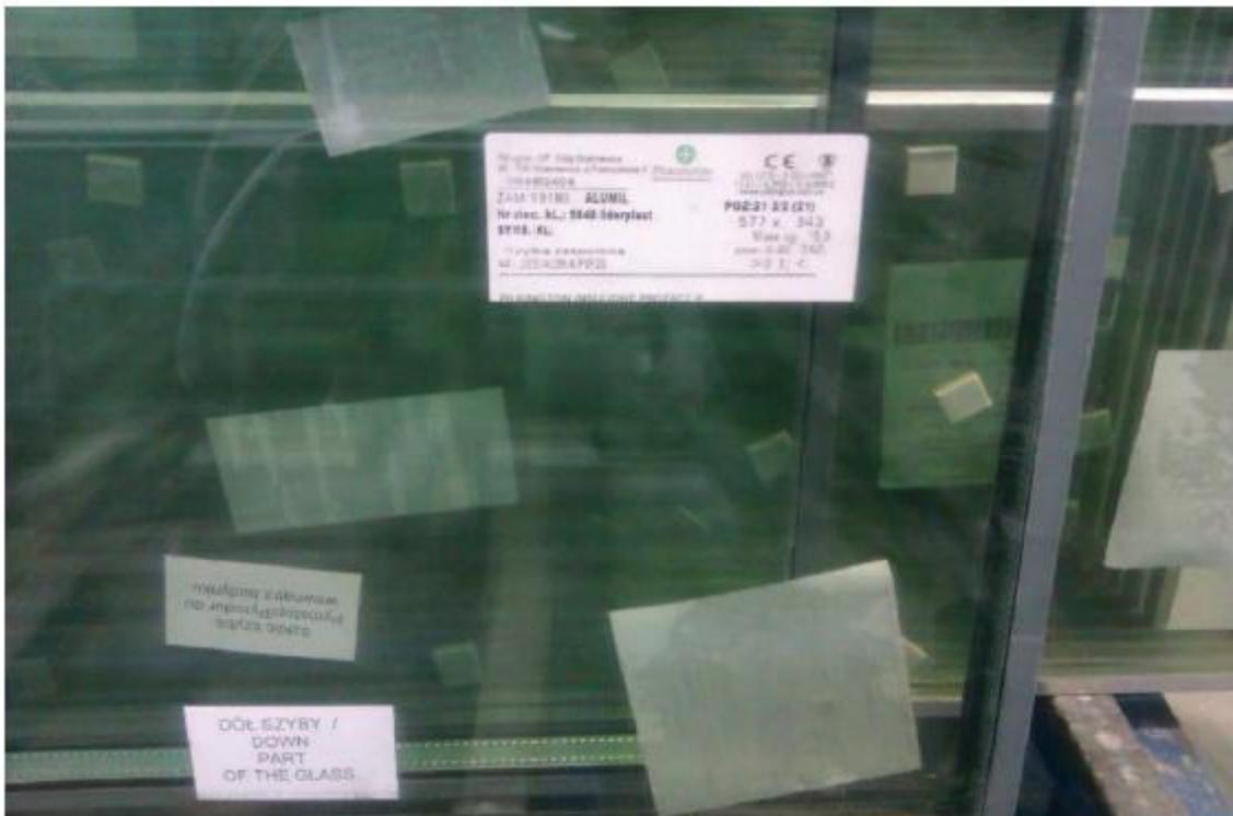
The edges of the glass are protected with aluminum tape. It is strictly prohibited to damage this tape because this will result in leakage of fire resistant gel and loss of fire-proof properties.
